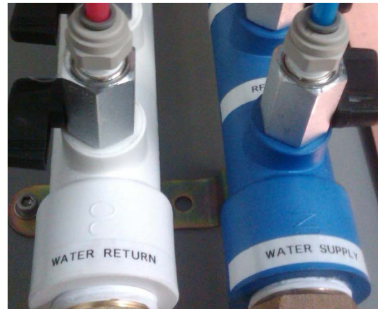
WATER MANIFOLD CONNECTIONS
